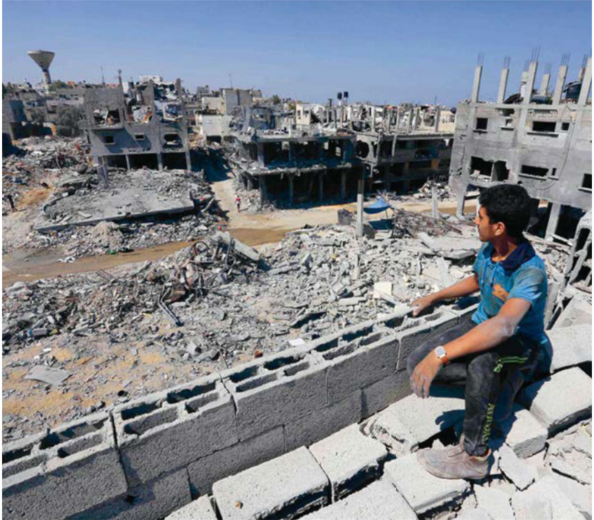
Photo 9. Structural damage caused by explosive munitions in the northern Gaza Strip, August 2014 (photo credit: APA Images).
